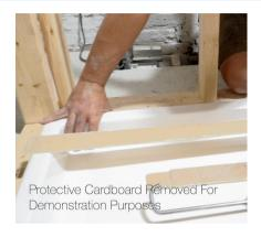
**7.** The shower base comes with a flange kit for proper fitting and to prevent water leaks.
