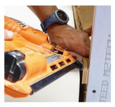
**12.** You may require shims for a tight fit for the flanges. Use as many cardboard shims as needed to secure a tight fit. Then, tack them into place.
