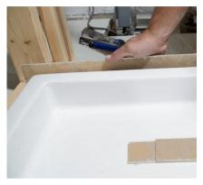
**9.** Place the flange carefully against the back side of the shower base making sure you have a good seal. Overlap the edge slightly so the flange will seal correctly at the corners.
