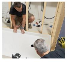
**3.** Push the shower base carefully in leaving about a half inch clearance from the back wall to accommodate flanges.
