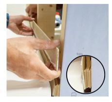
**15.** Slide the shims carefully into position leaving one to one and a half inches of clearance from the top of the base.
