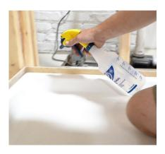
**18.** Always keep a clean work area and make sure to clean up residual silicone seepage with denatured alcohol.
