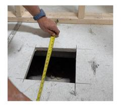
**1.** Measure carefully to determine the plumbing position and create plenty of access.
